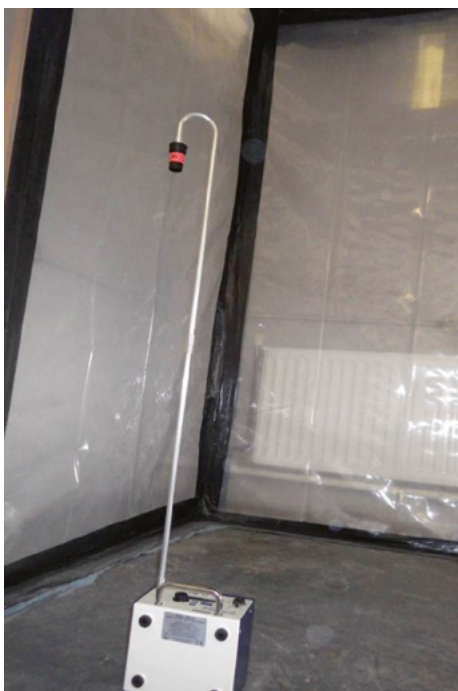
Figure A5.6 Air sampling during clearance
