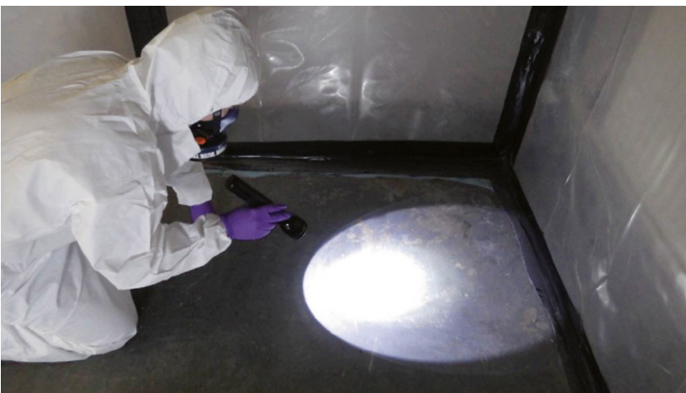
Figure 6.4 Analyst carrying out the thorough visual inspection
