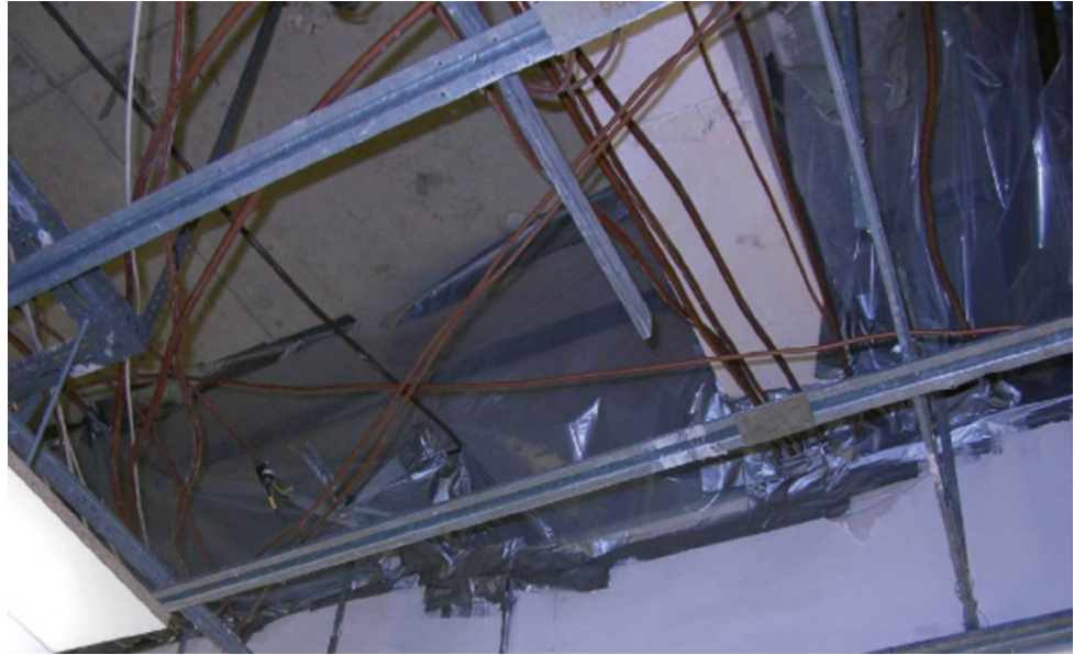
Figure A5.4 Void photo showing locations and extent of surfaces, cables and other items that need to be visually inspected for dust and debris
