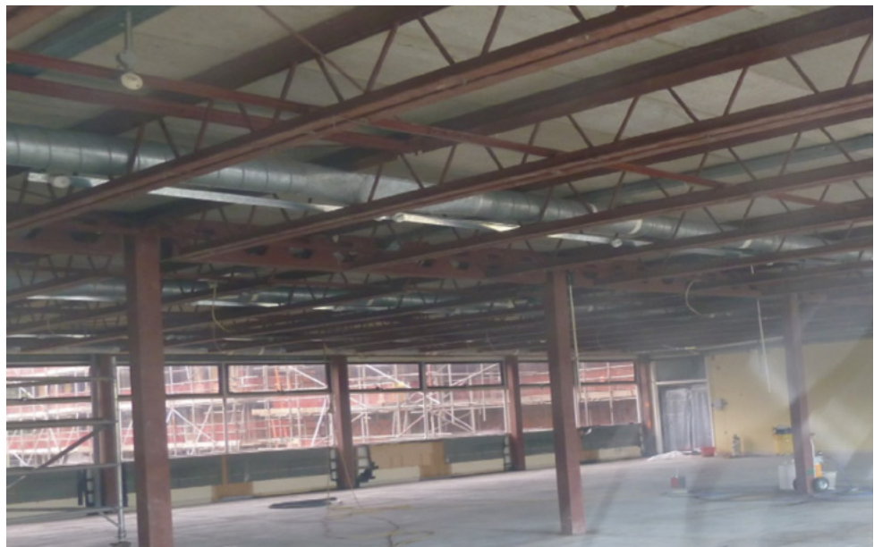
Figure 4.4 Photograph of a site where dust is likely to be present on high-level surfaces
